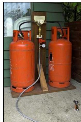
To get started I built a small gas fired kiln, gas being supplied by two 19 Kg cylinders with an automatic swap-over valve. and started exploring slip casting, hand building, glazing, and Raku, allowing me to work through the whole process, discovering not only the shapes, forms and textures that can be achieved with clay, but also the wonders of glazes and the colours that can be generated through varying the firing process.
